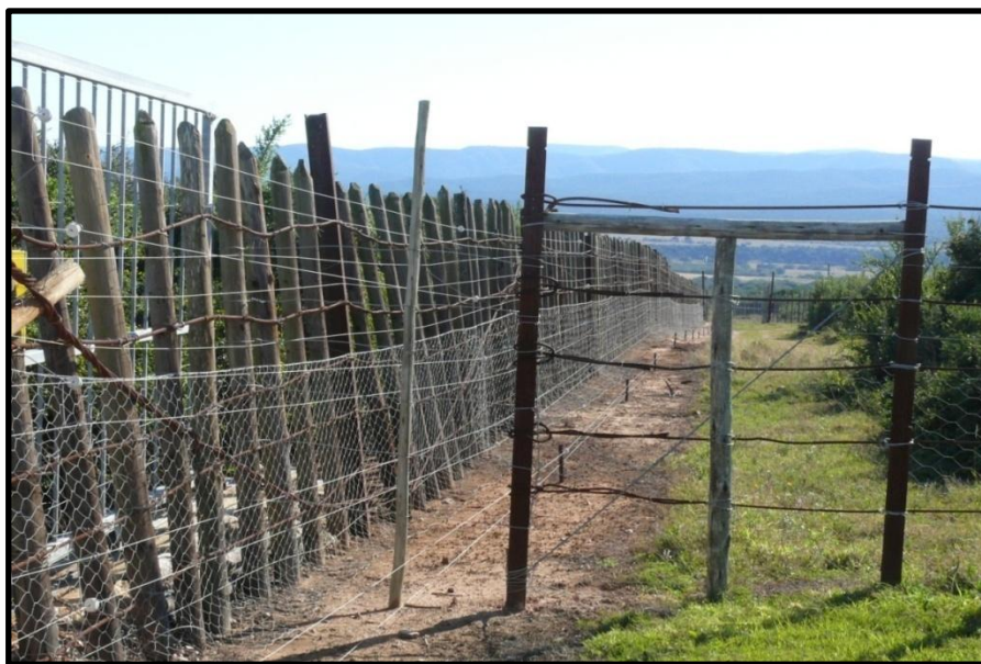
Fig. 9: The Armstrong Elephant Proof Fence at Addo National Park, near Port Elizabeth, in South Africa. This mechanical barrier, constructed in 1954 by Graham Armstrong, from discarded pieces of tramline, has stood the test of time in containing a growing population of elephants within the park.
